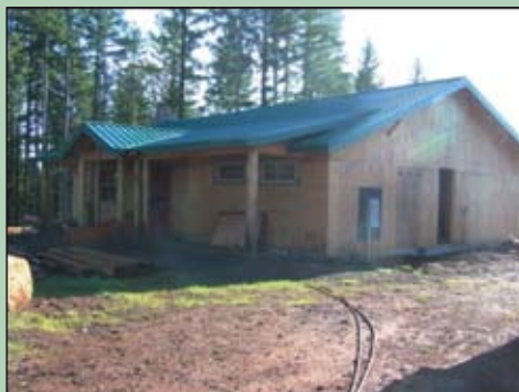
Front of the new classroom with windows in place.
