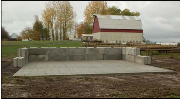
A bioswale is planned to handle runoff from the concrete composting pad.
