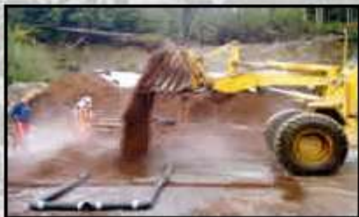
Laying a base of wood chips on the aeration piping.
