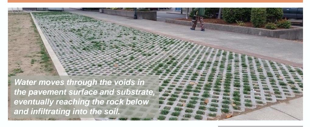
Permeable pavers, like the ones pictured above, are a cost-effective solution that provide pavement structure with water quality benefits. City of Coos Bay Public Works Department opted to install permeable pavers on a 15 ft. setback of Central Avenue to accommodate street vendors for the farmers' market. Porous pavement technologies have evolved significantly over the past two decades; when properly designed and installed, the pavement can effectively manage stormwater with low maintenance.
