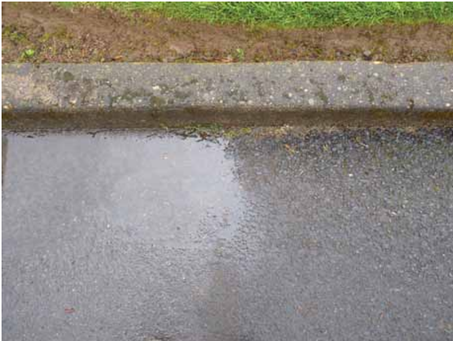
Porous asphalt pavement next to impervious pavement.
