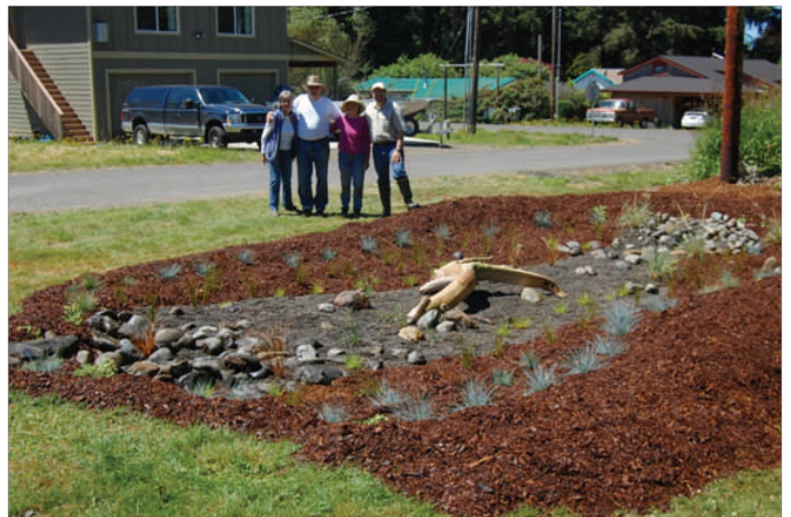
Above: Volunteers Chris Bolger, Larry and Andrea Goss and OSU Water Resources Extension faculty Robert Emanuel pose in front of the finished rain garden on July 1.
