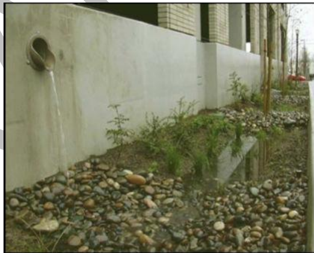
Figure 4 Filtration planter built into parking garage (NYSDM 2007)
