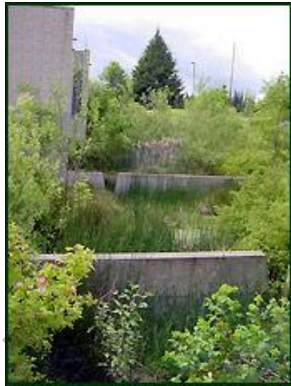
Vegetated Filter Strip, Portland, OR (Icrep 2008)
