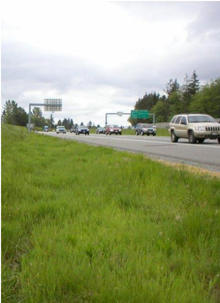
Vegetated Filter Strip along Highway (WDOT 2009)
