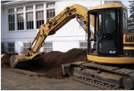
Figure 10A. Mix compost into the soil as deeply as possible. Add about 1/3 compost by volume. For large areas or areas with compacted soil, consider heavy equipment.
