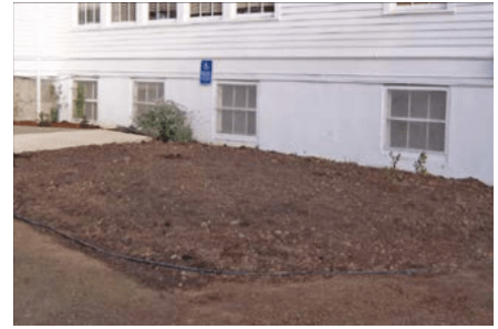
Figure 10C. The landscape bed ready for planting.
