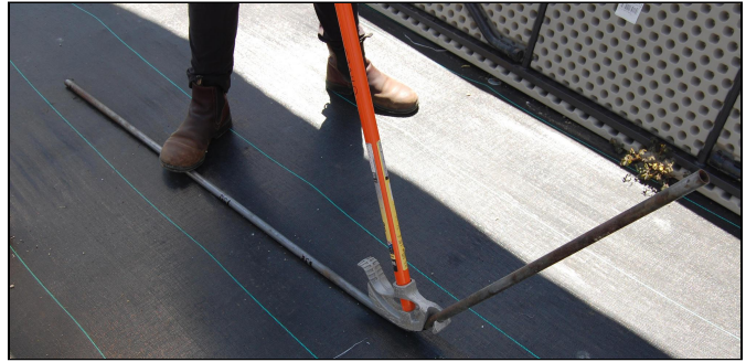
Figure 9. Use a conduit bender to shape galvanized conduits.
