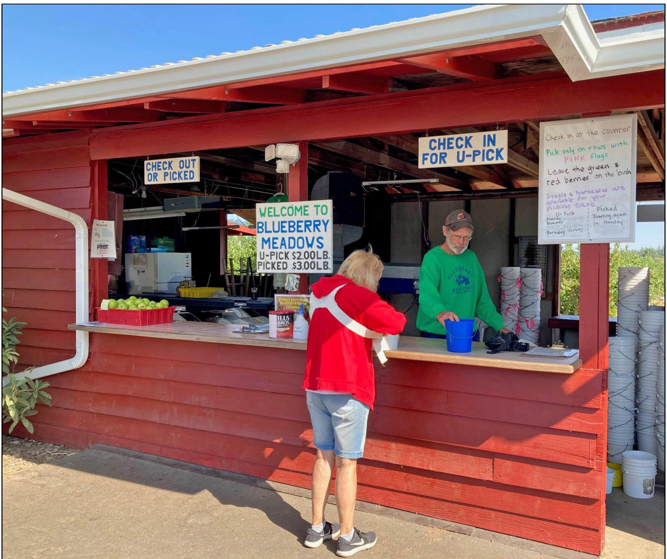
Depending on their use, structures such as farm stands must be built in compliance with county building codes.
