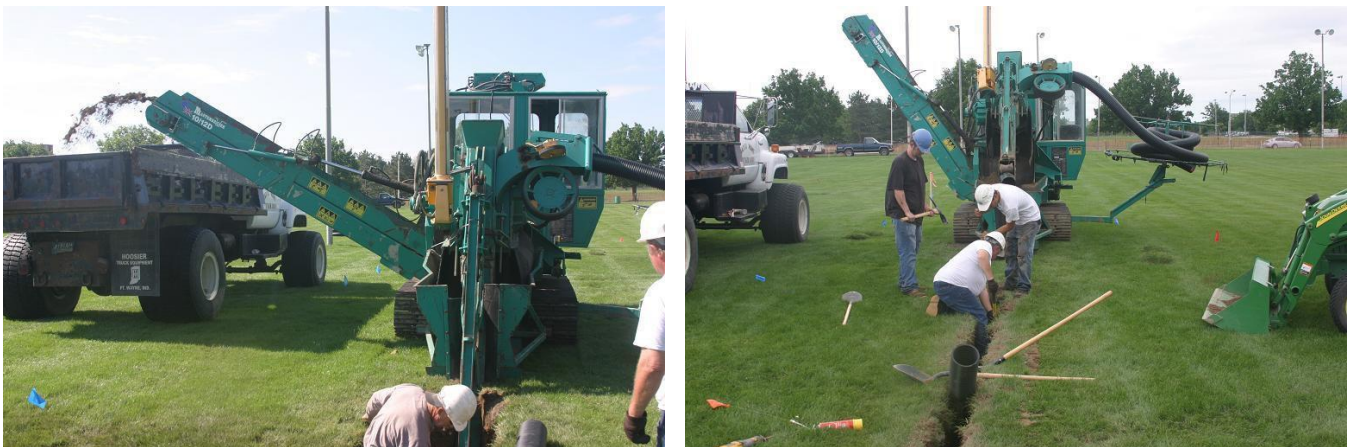
Figure 3: Drainage trenches (6 to 8 inches wide) being cut using a laser-controlled machine.
