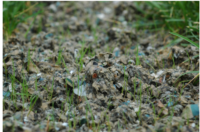
Figure 10. Hydroseeding with grass seed and approximately 1,200 pounds of fiber mulch per acre has been most successful in preventing the blowout of seed and sand.
