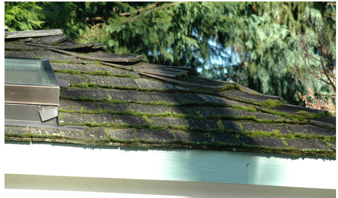
Figure 5b. Moss builds up on the thicker cut ends first.
