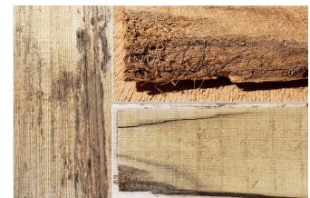
Figure 4a. Dark-pigmented fungi color the surface of these cedar shingles.
