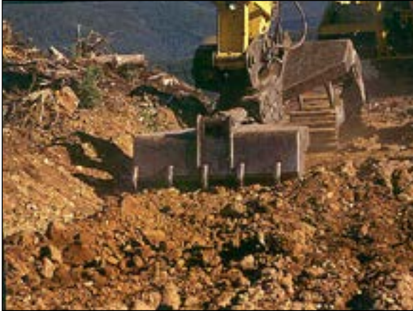
Figure 5.18. Tillage of a temporary road by using an excavator.
