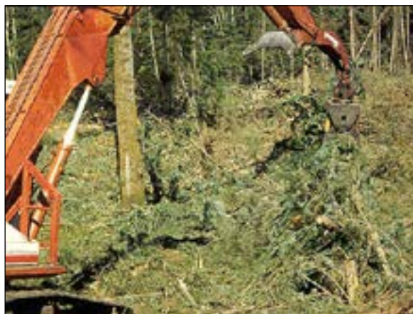
Figure 5.23. Place tops and limbs on the traffic lane and walk on harvest residuals before significant soil disturbance occurs, particularly on more sensitive soils.
