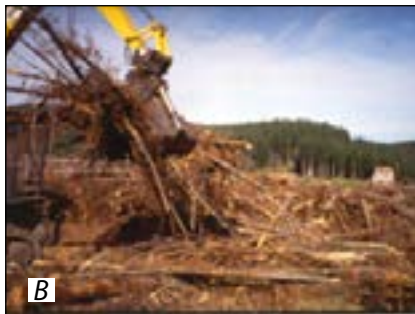
Figure 5.19. Replacement of (A) topsoil and (B) organic matter (logging slash) during rehabilitation of a temporary logging access road.
