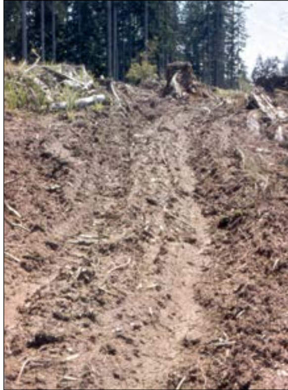
Figure 5.17. Deeply rutted Class 3 soil disturbance with the potential for erosion and movement of sediments into streams.
