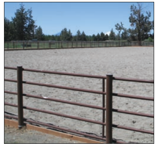
Footing material, such as this coarse sand, can be added to a drylot to provide a dry, stable surface. Other options for footing include gravel or shredded wood.
