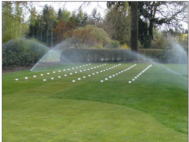
Figure 4. Catch cans can be used to evaluate the water delivery rate of a sprinkler system.
