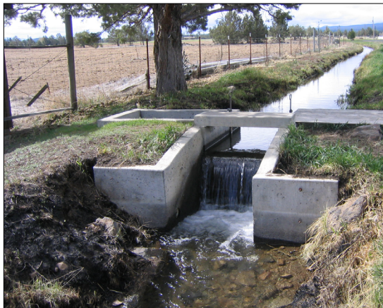
Figure 2. Irrigation districts often use a weir (a concrete or masonry structure constructed across an open channel) to measure water flow and divert water to patrons.
