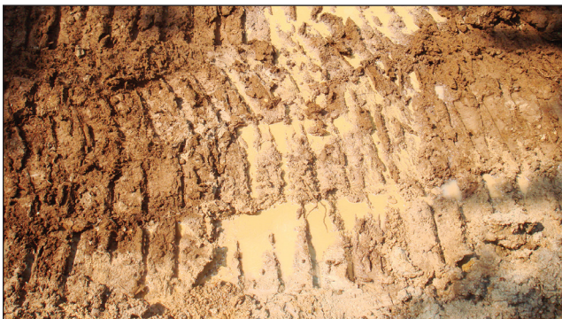
Clay deposits and water seepage immediately after excavation are good signs; clay helps hold water in the pond, and the seepage will help keep it full during dry periods.
