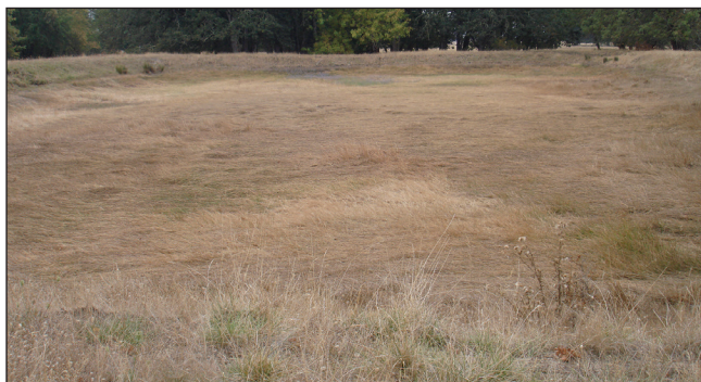
Porous soils and a lack of proper soil compaction caused this pond to fail before the summer was over.
