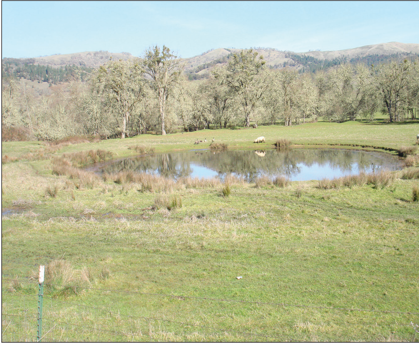
An excavated pond is a good choice for flat terrain.
