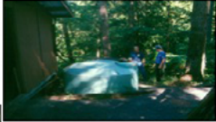
Cistern filled by rain water from roof
