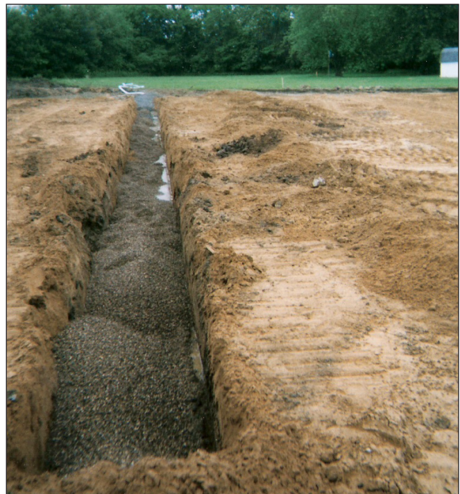
Photo: Howard’s Excavating, New Buffalo, Michigan Soakage trench under construction.
