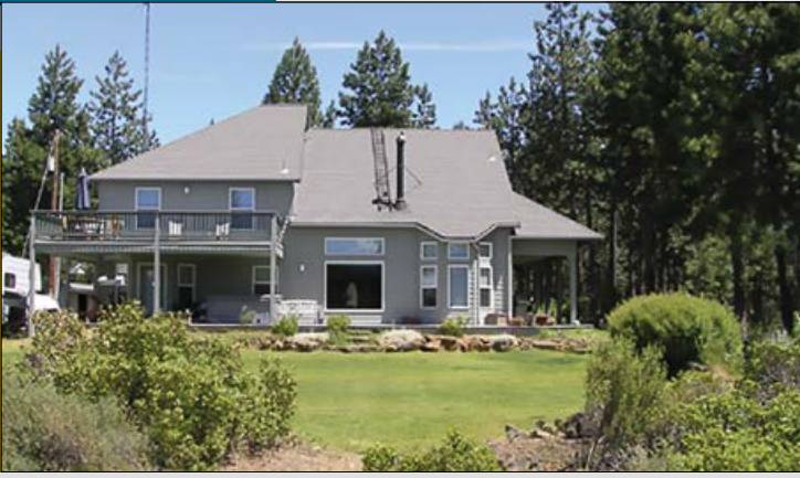
Figure 9. A well-maintained lawn can be part of a fire-wise landscape. Grass or alternative groundcovers serve as an effective fuel break. PHOTO: Stephen Fitzgerald, © Oregon State University
