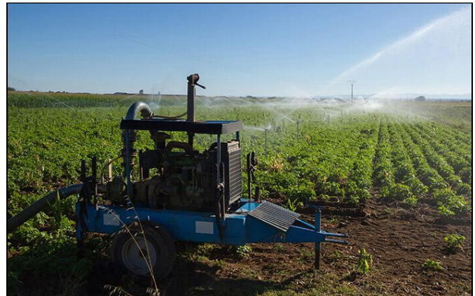
Figure 6. Diesel-powered irrigation pump supplying water to a sprinkler system in the field.
