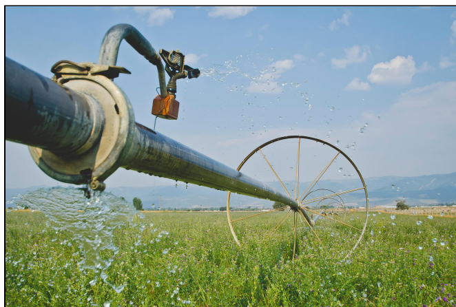
Figure 8. A wheel line irrigation system shows signs of poor maintenance.
