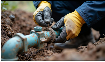
Figure 10A. Components of a solid set irrigation system. This is a manual valve connection along an irrigation pipeline.
