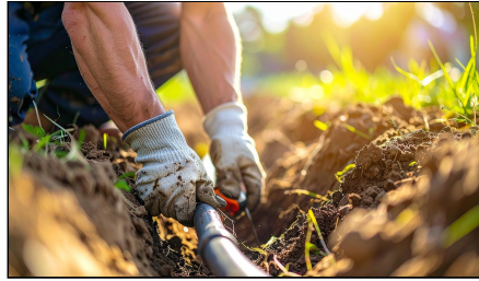
Figure 17B. Repairing irrigation pipelines and fittings prevents water loss.
