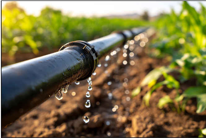
Figure 4A. A leaking mainline.
