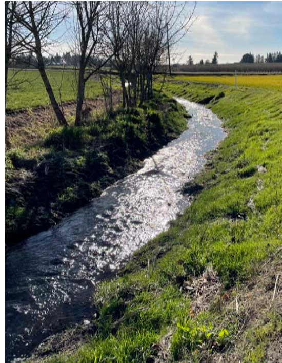
BRITTANY MILLS Sloped channel sides allow easier planting and vegetation maintenance while providing flow capacity.
